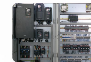
电器操控系统 Electric control system
